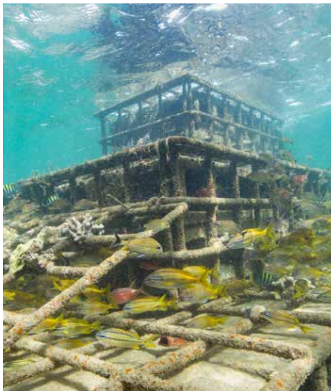
Pilot hybrid or 'artificial' reef structures, built with steel cages and filled with stones and cement, to protect a vulnerable coastline from strong wave action and the impacts from climate change, such as severe erosion © Tim Calver
