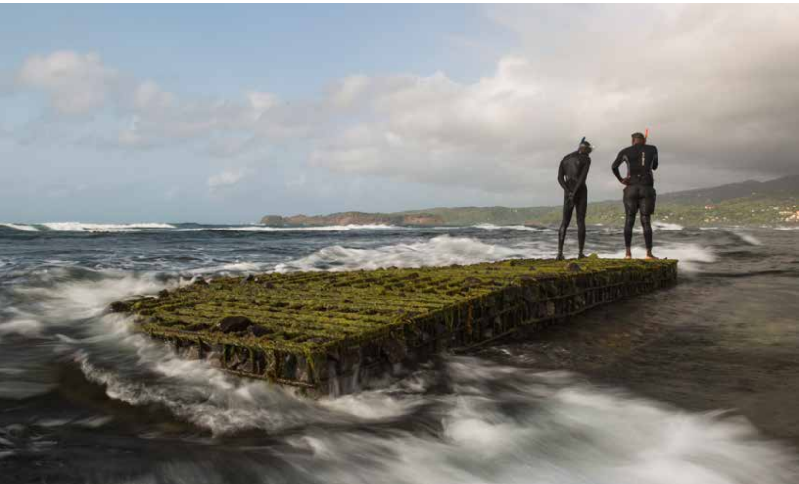
Two men stand atop an artificial reef in Grenada. The structures protect coastlines from strong wave action and reduce the impacts from climate change, such as severe erosion. © Tim Calver
