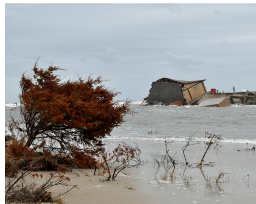
FIGURE 12. BREACHING OF HATTERAS ISLAND DURING HURRICANE IRENE (FEMA NEWS PHOTO).
